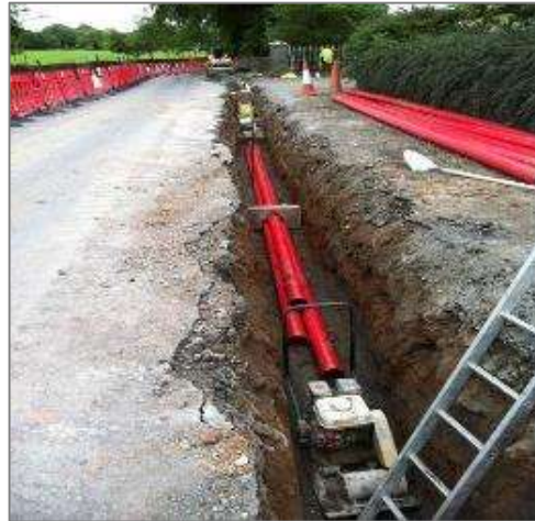
Figure 2 - 110kV Underground Duct Installation
