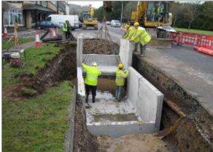
Figure 9 - Joint bay under construction (pre-cast)
