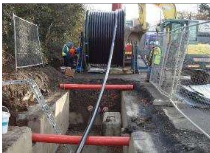
Figure 10 - HV cable pulling procedure (Typical drum set-up)
