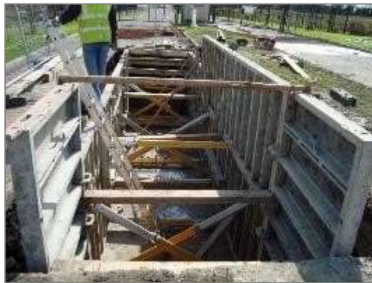
Figure 8 - Typical joint bay under construction (in-situ)
